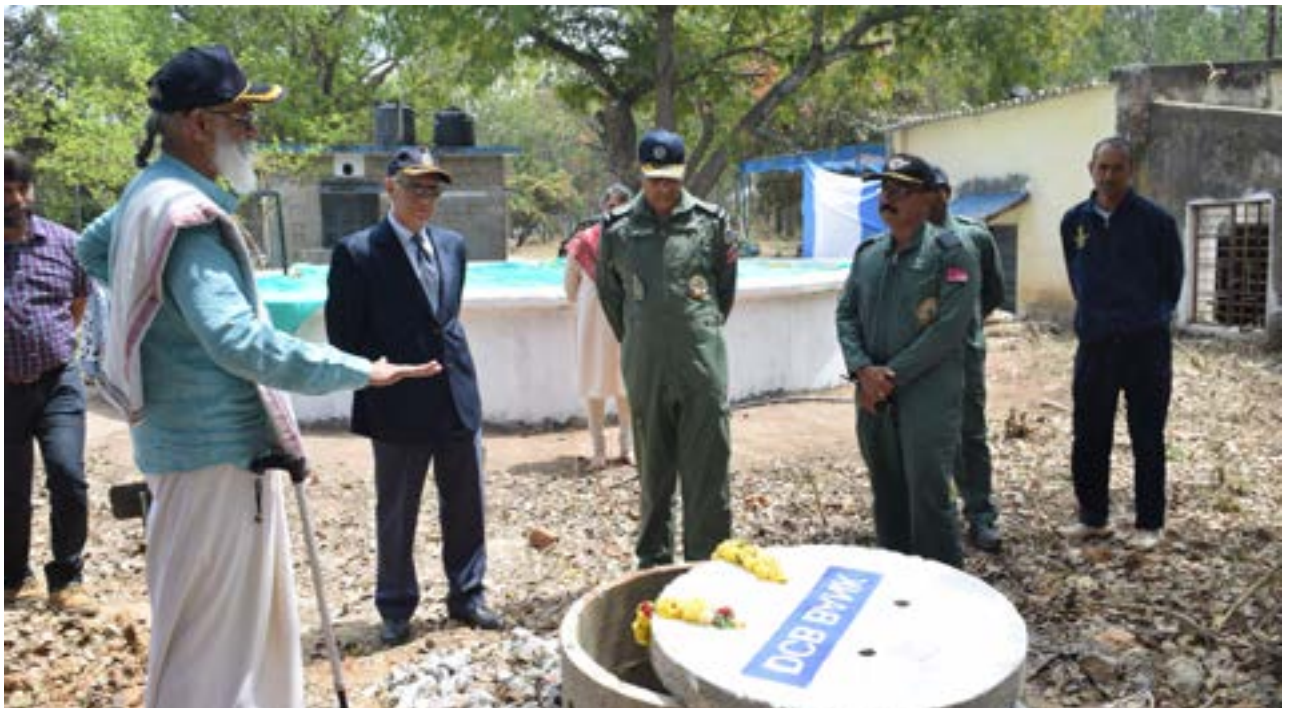
Water harvesting through Rainwater Recharge Wells, Bengaluru, Karnataka
